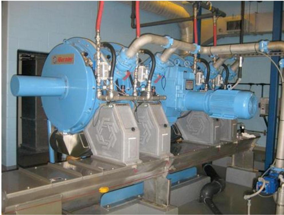
On July 9th the District made a major leap forward in the application of innovative wastewater technologies by bringing a new bio-solids press online at the Redondo Treatment Plant. Pictured above is the Fournier Rotary Press, which incorporates many of the technological advances in solids processing developed in the wastewater industry over the last fifteen years.
