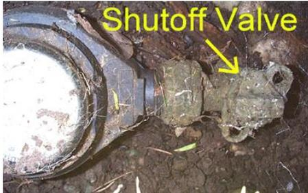
The water meter has a shut off valve in the box on the street side of the meter. The raised slotted angle valve again would be turned clockwise for closed and again care should be taken not to use extreme force when turning the valve as damage may occur. You will need a T shaped wrench for the shut off valve which may be purchased at most local hardware stores. You can use a crescent wrench and screwdriver as a makeshift T handle wrench. If you have any questions, call 253-946-5426.
