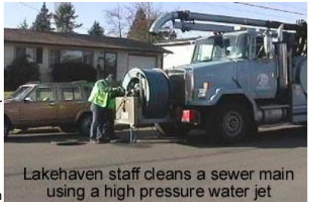
Lakehaven staff cleans a sewer main using a high pressure water jet
